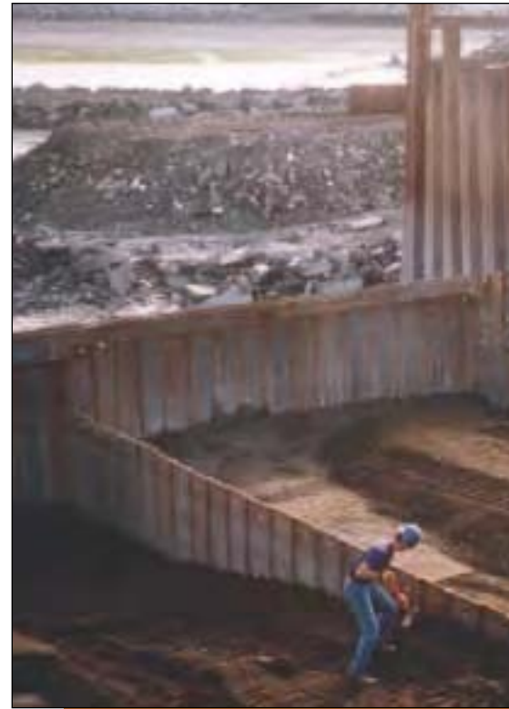
Open cell fill in progress
