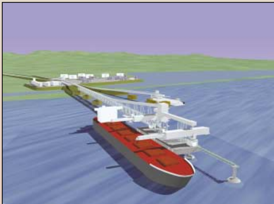
DeLong Mountain Terminal trestle and roadway extending to a deep-sea berth in the Chukchi Sea is shown in front of the existing dock. Courtesy Alaska Industrial Development and Export Authority.
