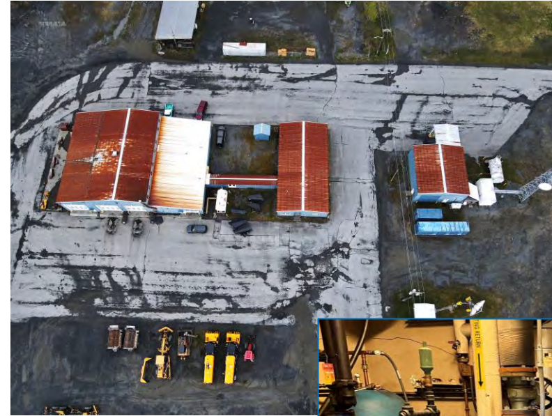
DOT&PF Valdez Complex Roof Replacement
