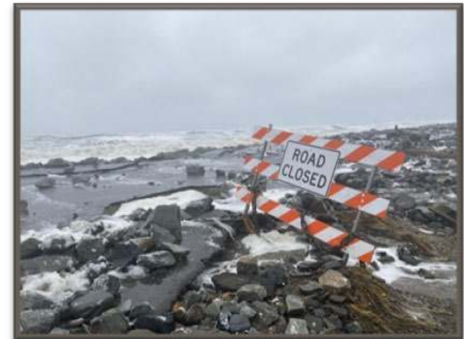
Overtopping after storm
