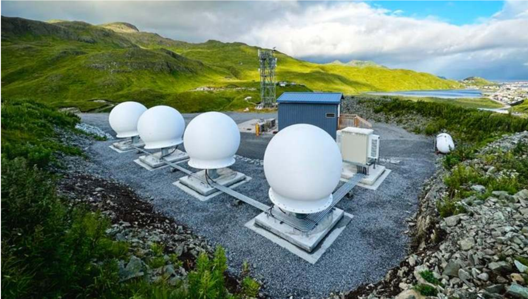
The first Starlink community gateway located in Unalaska, Alaska. Photo: SpaceX
